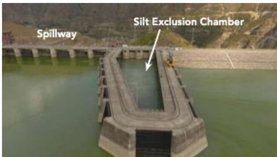
Figure III.1 - Pictorial view of Kol Dam decanting chamber in operation (Fig. 6c of Kumar and Singh (2022) with text annotations added). 142
