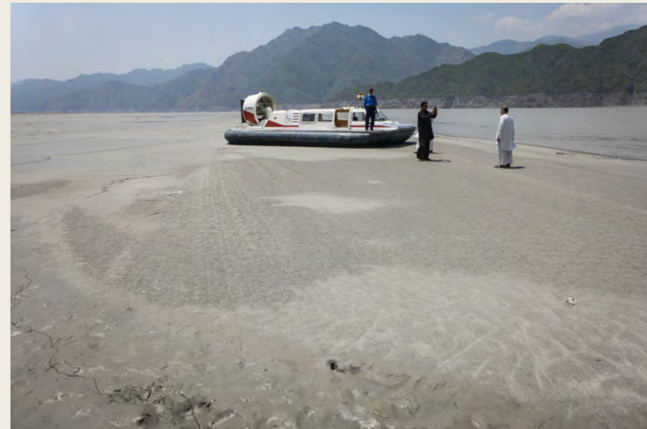
Top of the sand-silt delta advancing toward Tarbela HEP dam, Pakistan.
