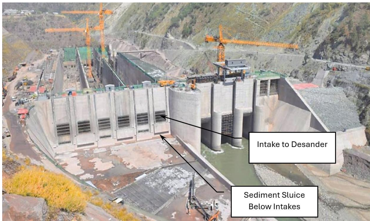
Figure 4.18 – Intake for the Neelum-Jhelum HEP showing sediment sluices below the intake 376
