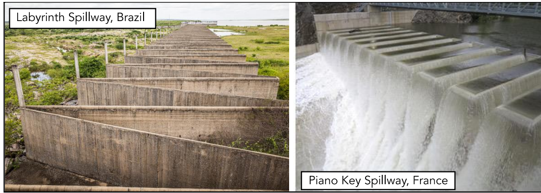
Figure 4.24 - Examples of Labyrinth and Piano Key spillways 385
