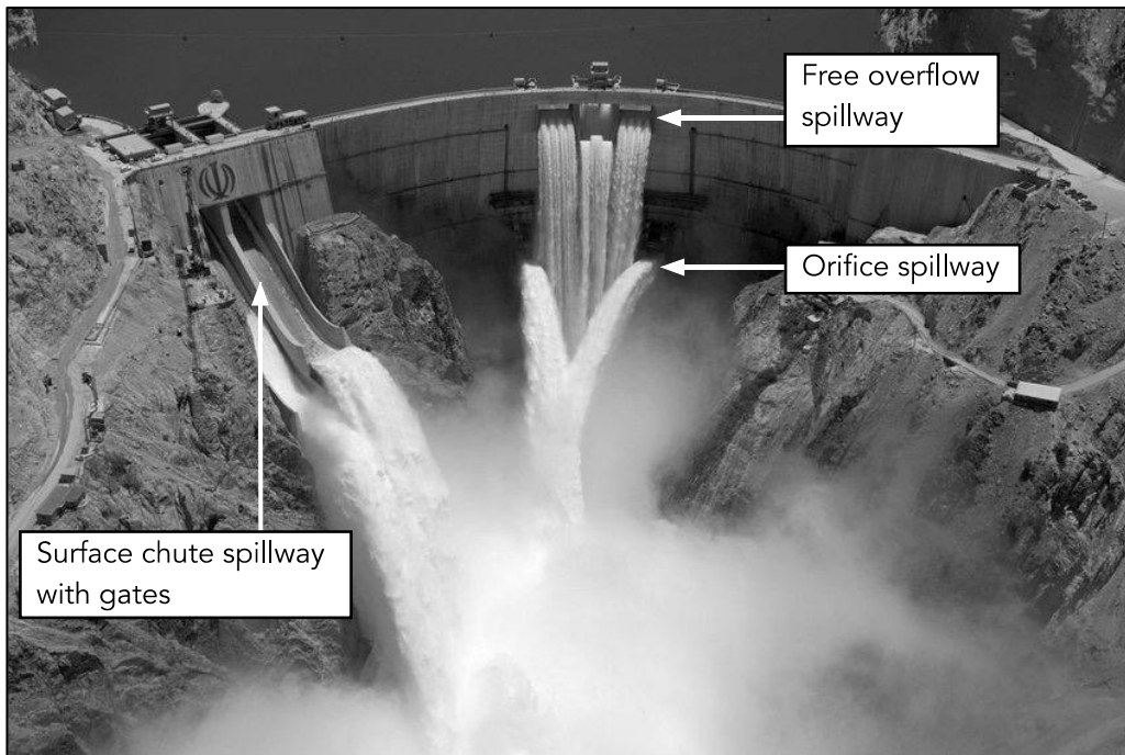
Figure 4.21 - Spillway at Karun III dam, Iran 380
