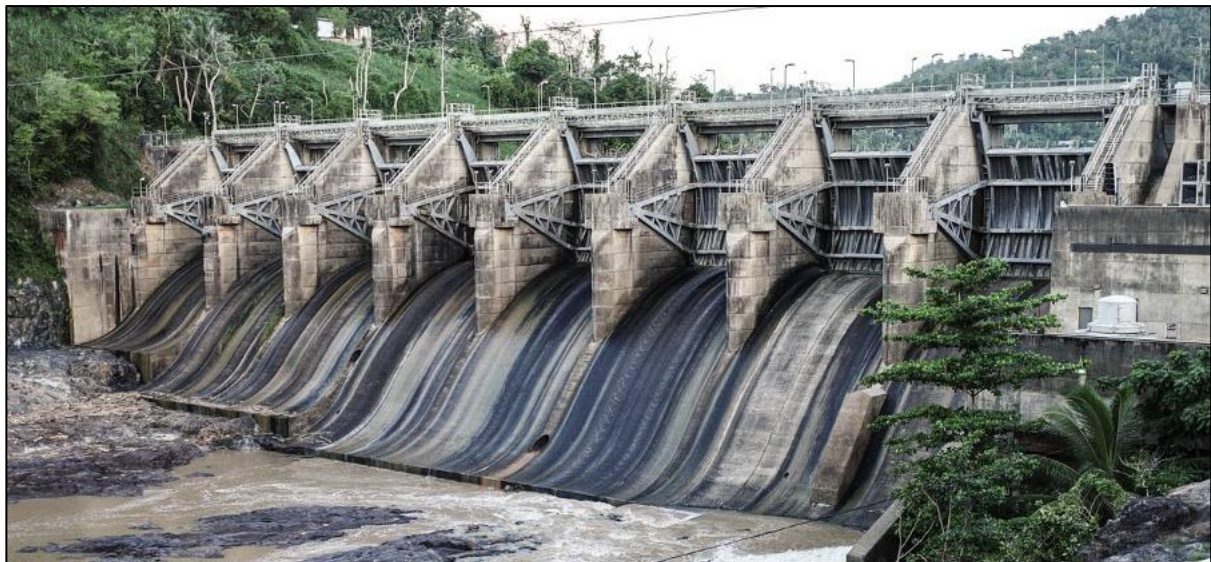
Figure 4.25 - Free-surface spillway with 10-metre-tall radial gates on the crest (Loíza, Puerto Rico, USA) 386
