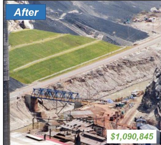
*South portion of plant with stabilized slag deposit in background (c. 2008).*
