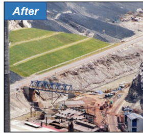
South portion of plant with stabilized slag deposit in background (c. 2008).
