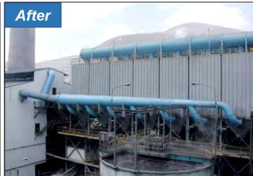
Lead Blast Furnace with dust collectors and enclosure (c. 2008).
